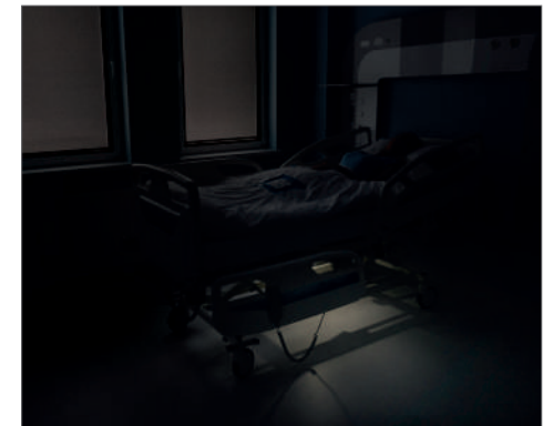
Ambient LED light under the bed.
